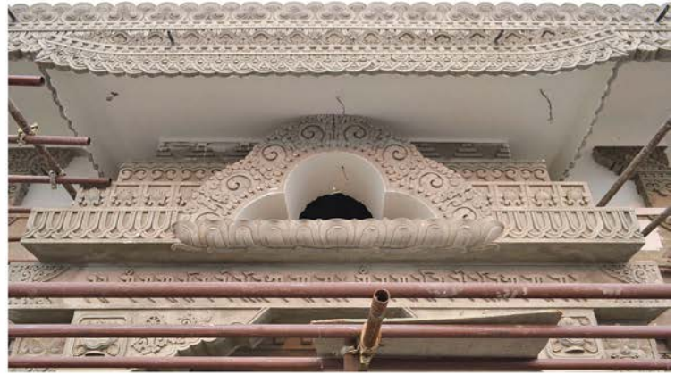
Figure 10. Recently Applied White Cement Putty on Underside of 3 rd Floor Curved Roof and Archway
