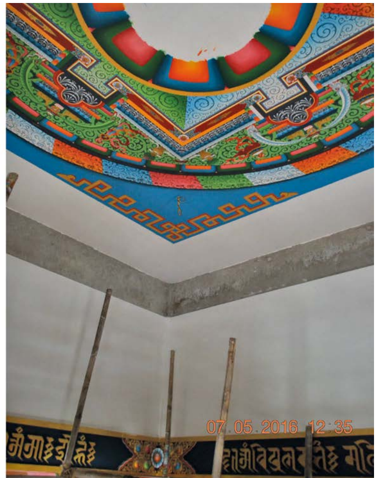
Figure 22. Partially Completed Central Roof Mandala Painting for 2 nd Floor Waiting for Installation of Roof Beam Decorative Blocks (see Fig. 12)
