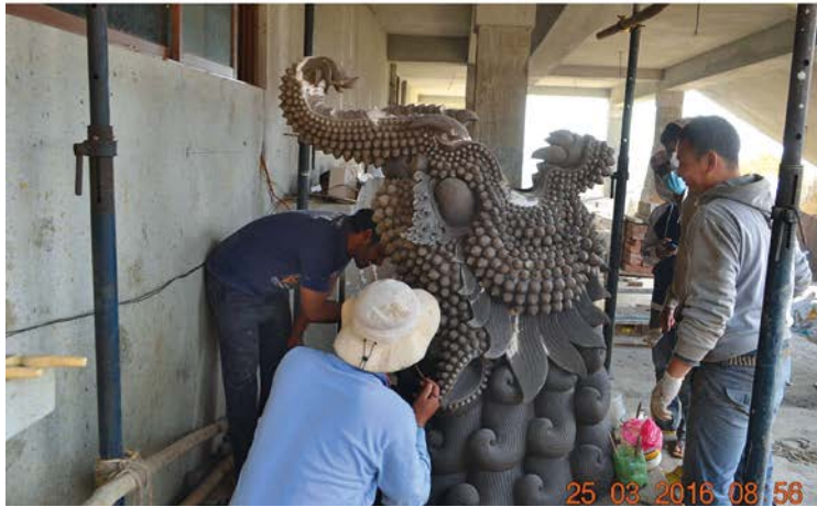
Figure 14. Model of "Chuzin" for Decorating Corners of 1 st Floor Curved Roof, Before Rubber Molding
