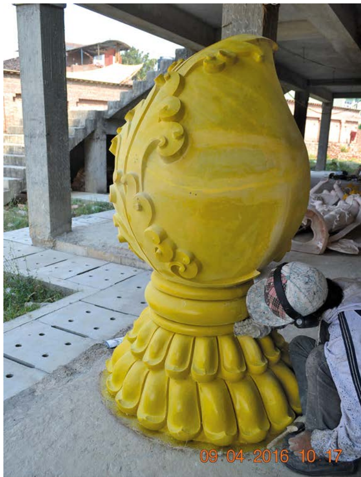
Figure 16. Pre-casted Jewel Tip for Decorating Corners of 2 nd Floor Curved Roof
