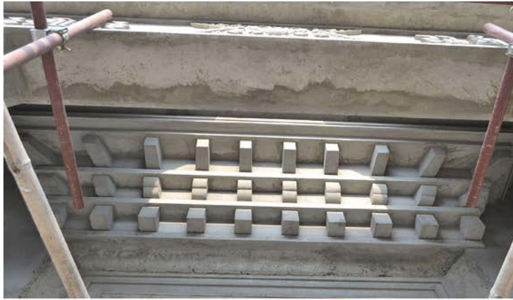
Figure 9. Close-up of Cement Decorative Blocks above the West Door on 2 nd Floor
