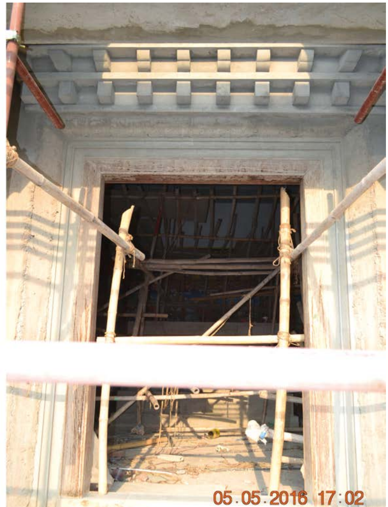
Figure 8. Recently Rough Plastered Decorations above the West Door on 2 nd Floor
